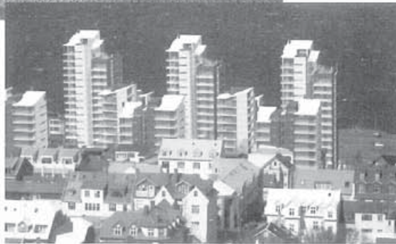
New housing project close to the city core
