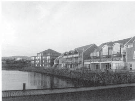
New housing built on a fill - "Marina". The houses are surfaced with corrugated iron as was the tradition in the "Old City".
