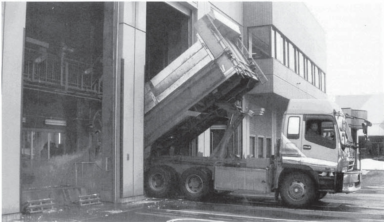
Sapporo Japan introduces snow into treated wastewater, which because of its heat, rapidly melts the snow.
