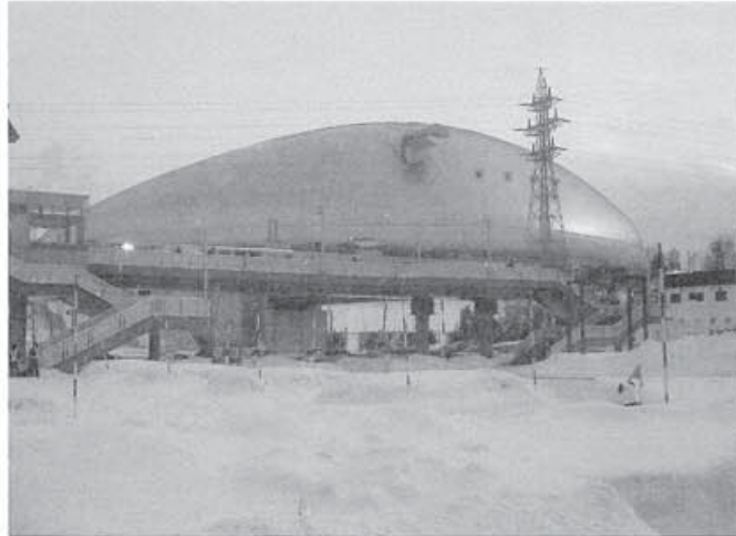
Sapporo Dome with snow shedding roof
