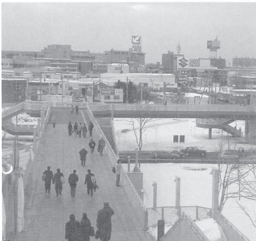
Elevated and heated walkways with yellow bricks and elevator/heated stairway at mid-right
