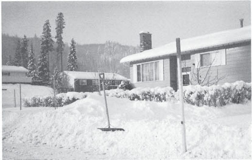
A snow shovel illustrates a typical windrow of snow in a residential driveway after a grader has passed following a light snowfall.
