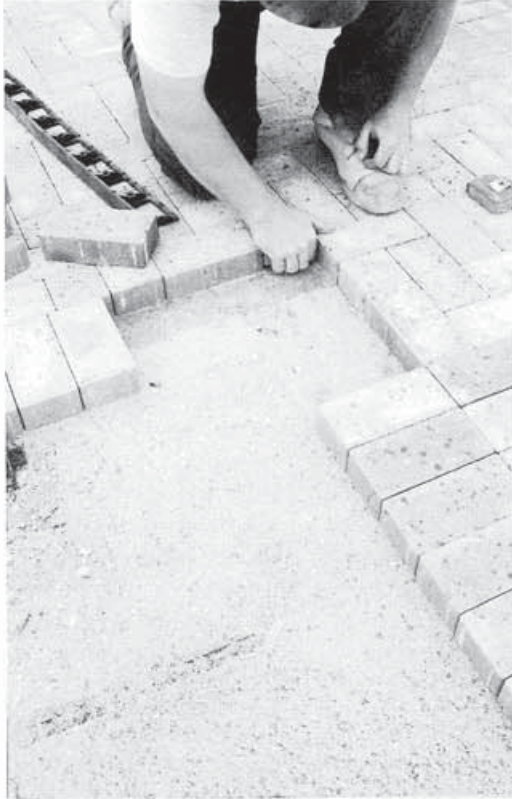
Concrete pavers can be installed year-round.
