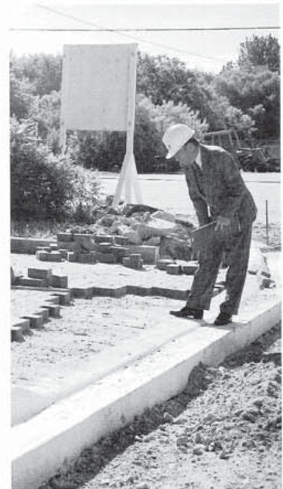
Brian Burton examines the installation of concrete pavers in London, Ontario.
